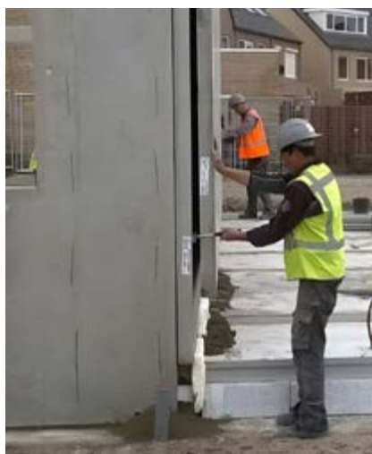
The AIRTIGHT® Air Stop during the installation of the party wall.
