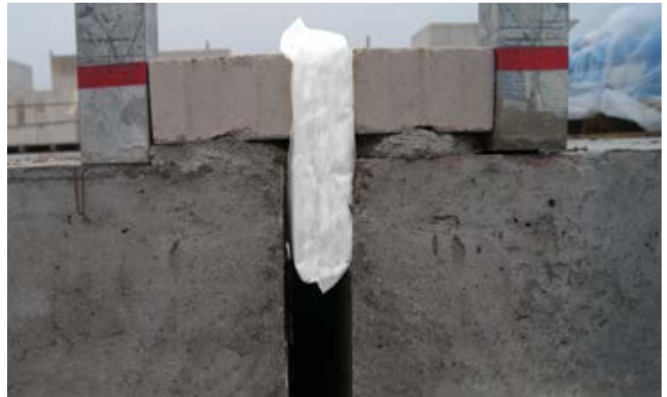
De AIRTIGHT® as an airtight seal between the party wall.
