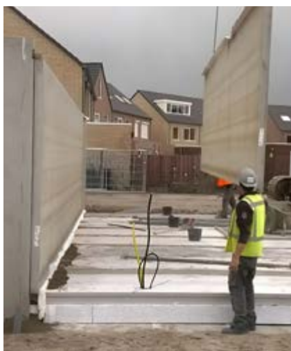
The AIRTIGHT® Air Stop during the installation of the party wall.
